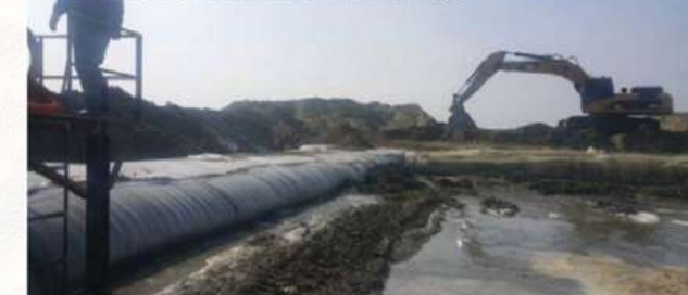
3. Sediment Settlement & Drainage
